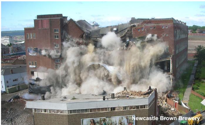
Controlled Group, the Yorkshire based Demolition Company collaborated with ASI for the first time in the UK and, the results were great. "The similarities between the predicted collapse and the actual collapse were impressive" said Controlled Structural Engineer, Rob Clarke.
